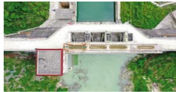
●龙虎水库大坝
