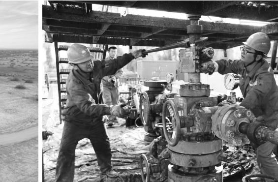
●对长期关停井实施检泵作业,使其“起死回生”
