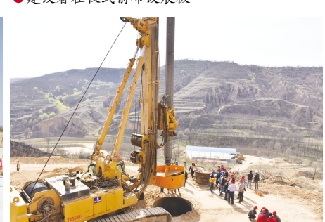
●旋挖钻成孔
